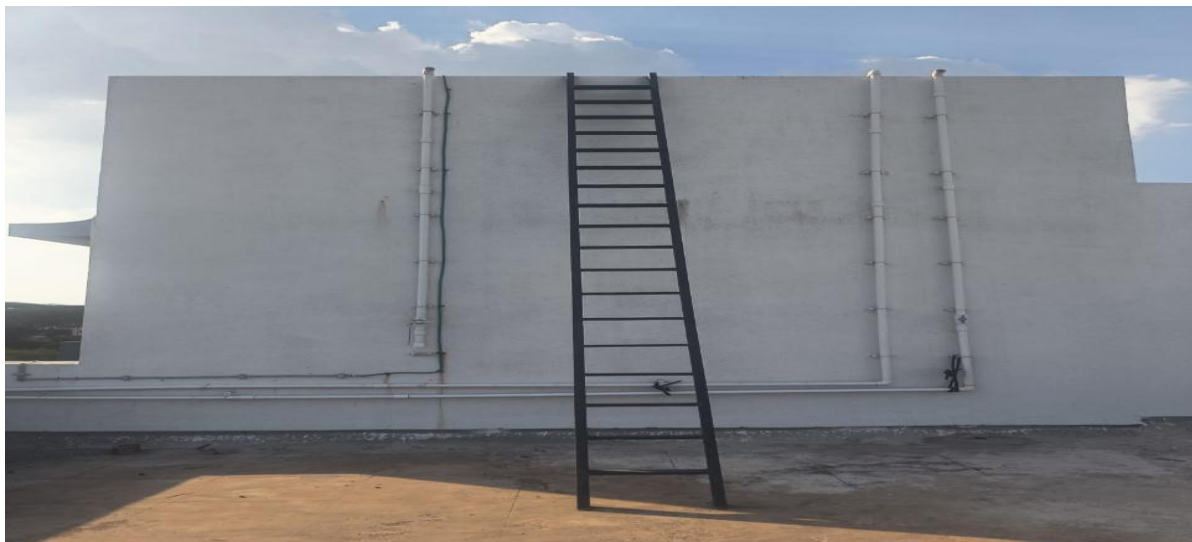
Water Tank For Hostel ( 10,000 Litre Capacity)
