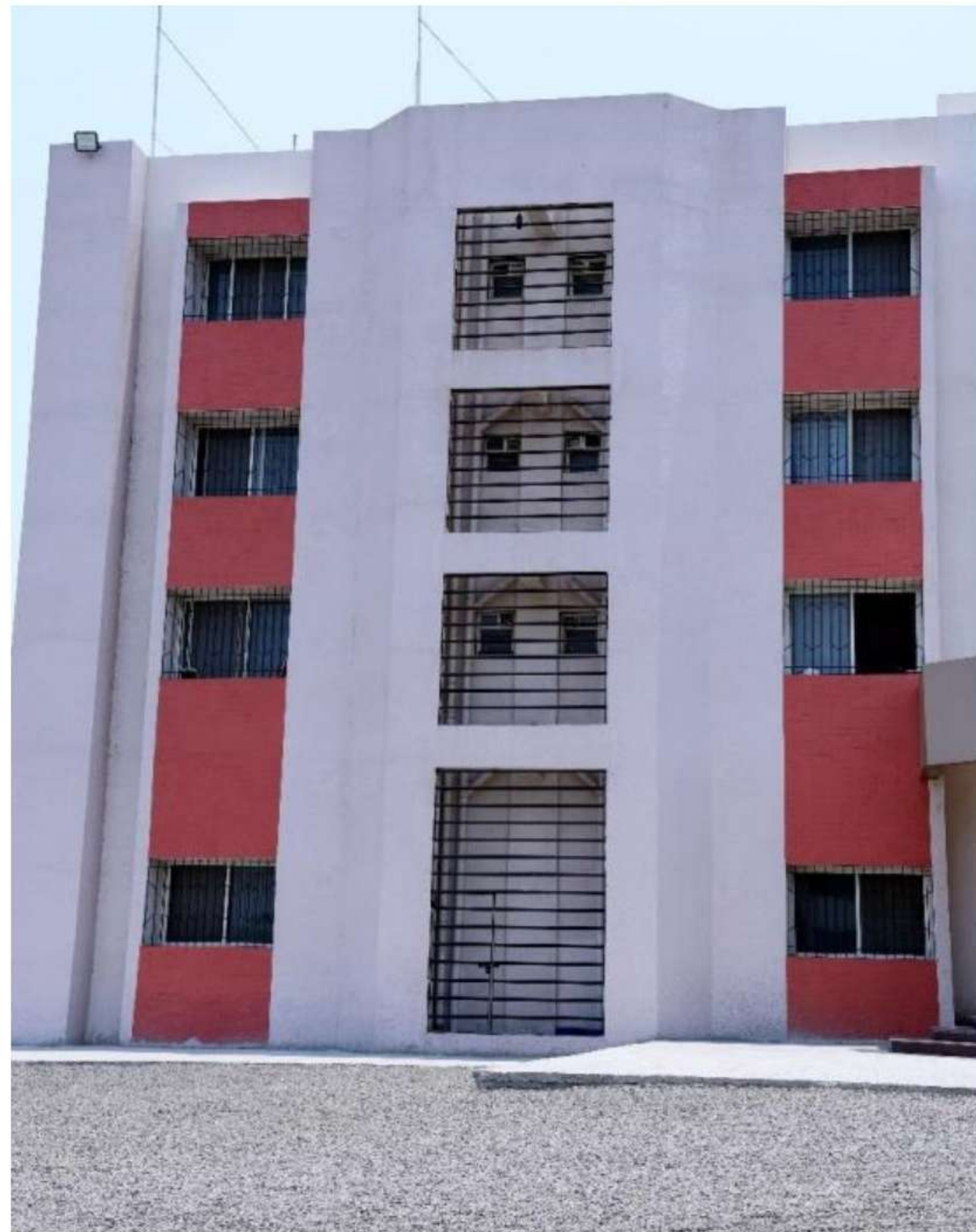
Rain Water Harvesting arrangement at Girls Hostel)
