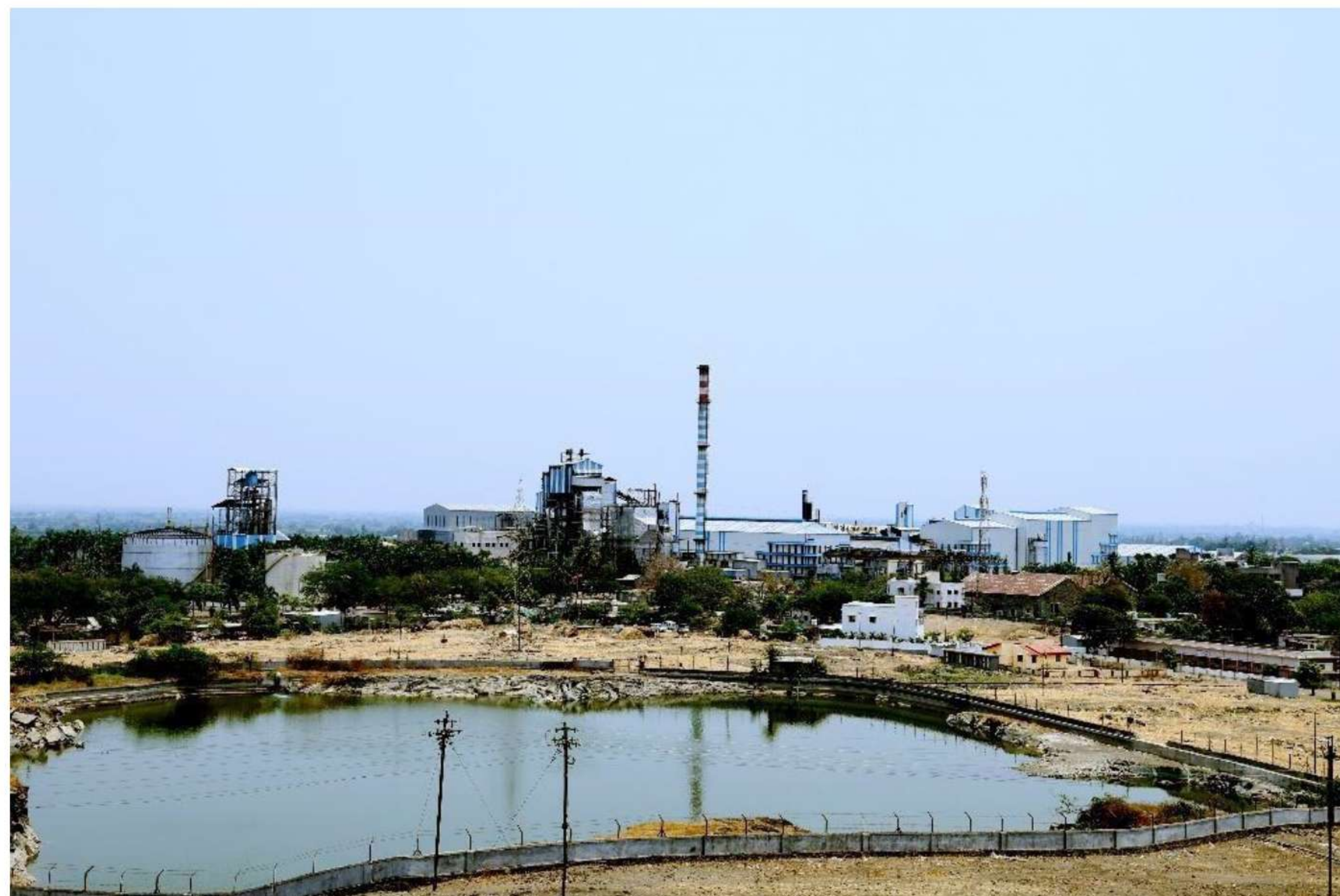
(Rainwater harvesting storage tank in the institute campus)
