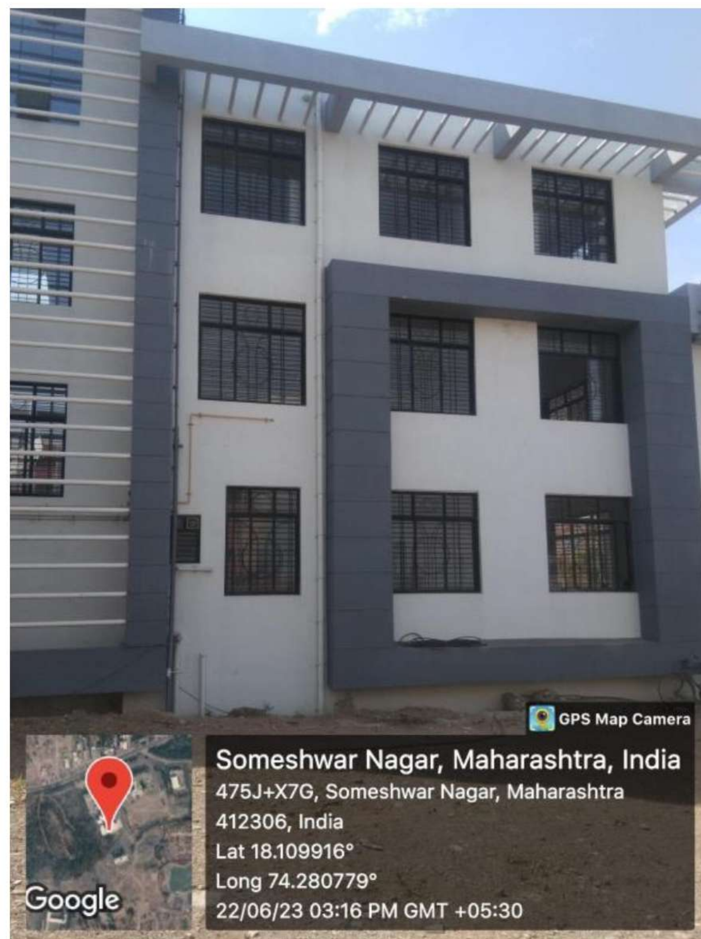
(Rain Water Harvesting arrangement at institute building)
